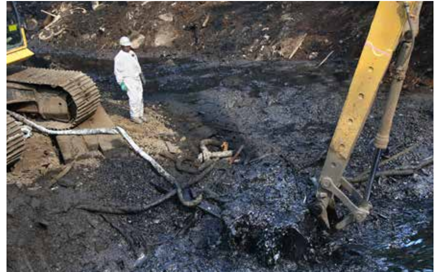
Toxic coal tar was removed from a section of the Creek during a 2006 remediation. Photo: Charles Denson.
